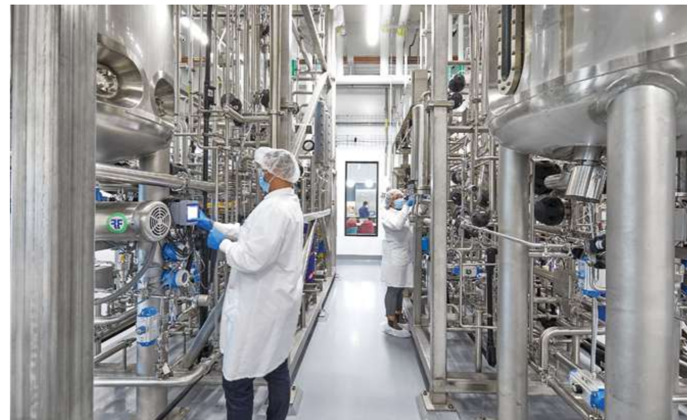
Upside Foods facilities. Photo Upside Foods
